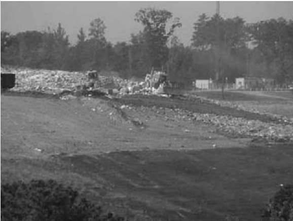
FIGURE 6.3 Trash Loaded and Compacted into a Landfill. 9
