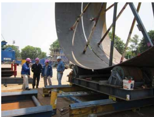
The Teesside facility will utilise Alter NRG plasma gasification technology Credit: Alter NRG
