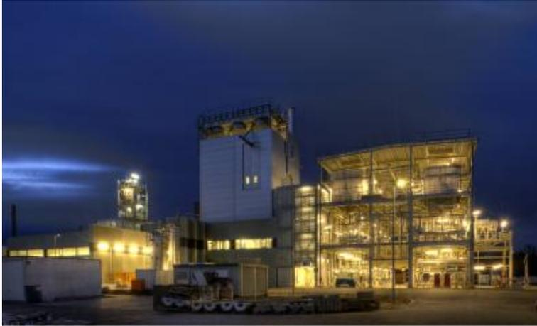
This shows the bioliq plant at the KIT: in a multi-stage process, high-grade synthetic fuels are produced from straw and other biogenic residues.
