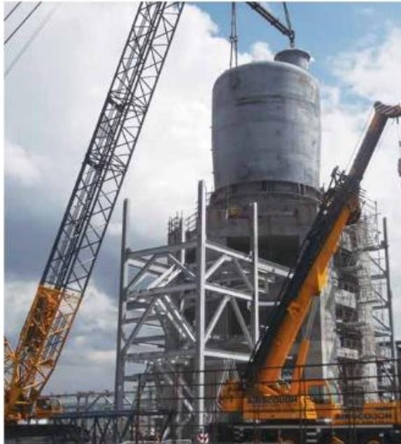
The heart of the process is the plasma gasifier that will daily convert 950 tonnes of municipal solid waste to syngas, which will then be consumed in the power generation section. In May, the site took delivery of the main gasifier vessel which was transported carefully from the Tees River to site along three miles of narrow local roads.
